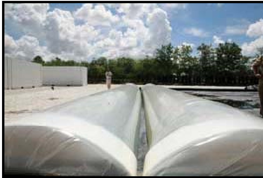
Algenol Biofuels Inc. algae to ethanol test facility in Florida
